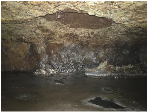
View of inside septic tanks – note deterioration of concrete
