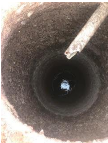
Effluent in seepage pits is a sign of future failure
