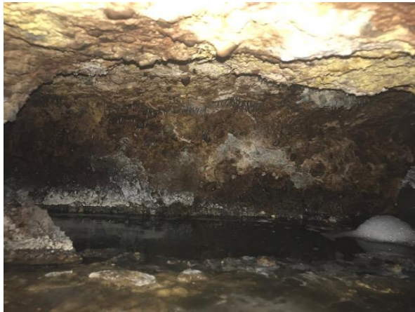
View of inside septic tanks – note deterioration of concrete
