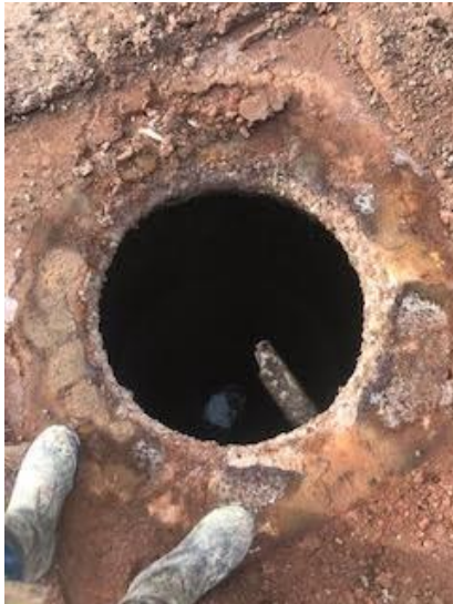
Effluent in seepage pits is a sign of future failure
